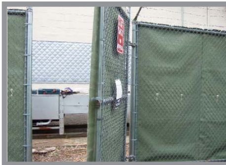
Panels were made for two of the walls of this enclosure, with a separate panel for the door.
