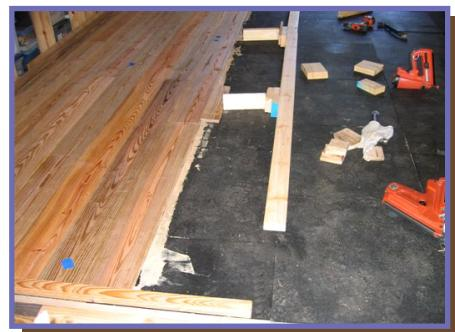
*It was very important to get these floor boards to stay very tight together. The 2 x 4 shown here were screwed through the Acoustik, into the subfloor to provide a strong, stationary point. Pressure was then applied using the other pieces of plywood pushing the boards tightly together until the adhesive cured.*
