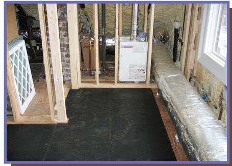
The seams of the Acoustik are staggered like bricks.
