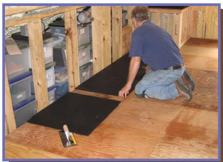
It is important to use a marine grade or exterior grade T&G subfloor so that moisture doesn't cause expansion.
