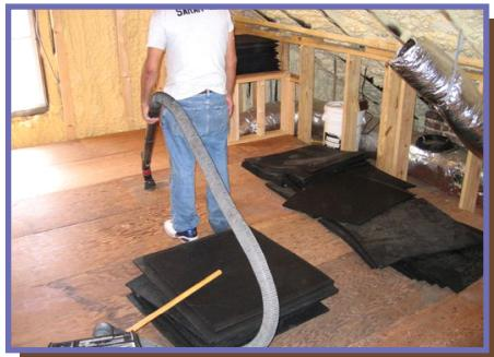
The floor was raised with plywood to hide the HVAC system for the house as well as to offer a flat surface for a subfloor.
