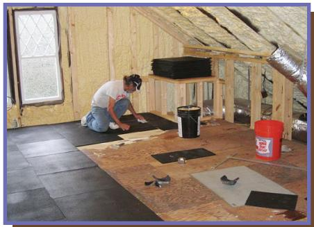
Acoustik underlayment is adhered to the new subfloor with our DA-5 two part adhesive. This adhesive has bits of recycled rubber in it and is installed onto the subfloor with a 3/16" notched trowel. The ridges of adhesive are an important part of the overall performance of the floor system. It will help decouple the rubber from the subfloor and offer a different rate of deflection to help absorb impact energy.
